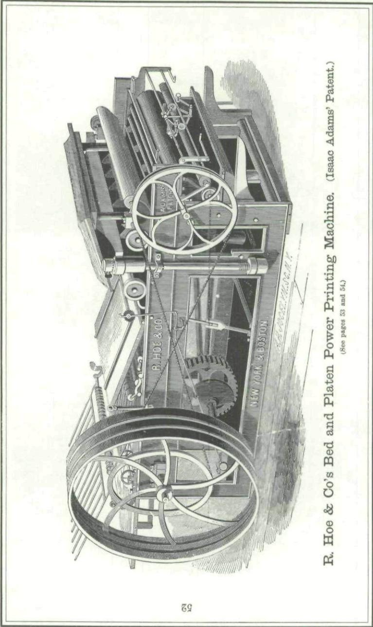
R. Hoe & Co's Bed and Platen Power Printing Machine. (Isaac Adams' Patent.)
