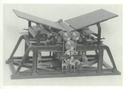
PLATE III.—Patent Office model of the 'Pony' Double Cylinder Press. (Courtesy of the Smithsonian Institution.)
